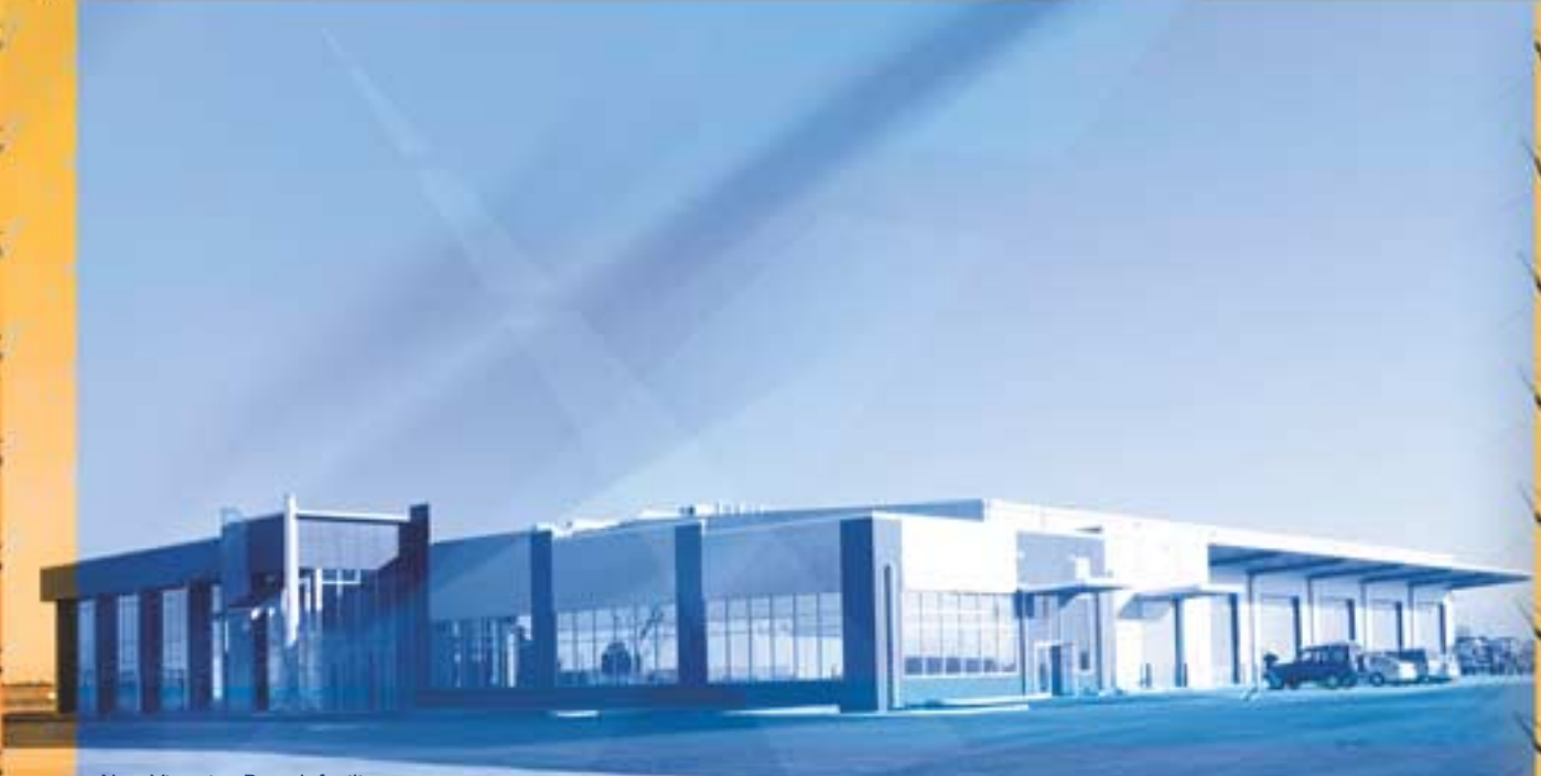
New Victorian Branch facility at Derrimut completed September 2002
